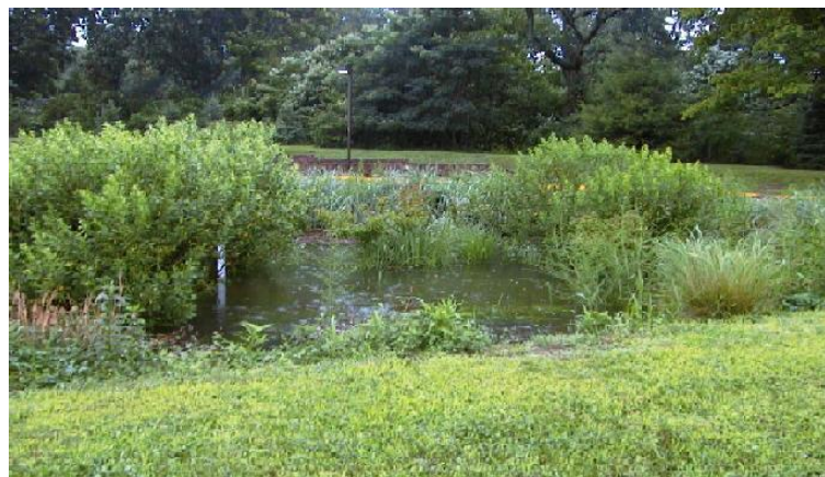
Villanova Bioinfiltration Traffic Island following a storm event
