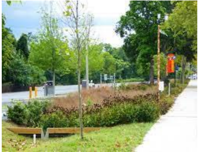
PWD Bioinfiltration GSI
